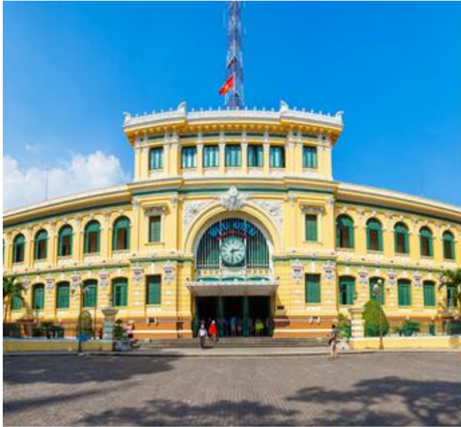
Central Post Office
